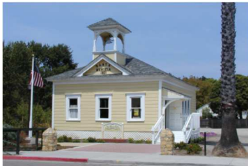
SANTA MANUELA SCHOOLHOUSE
